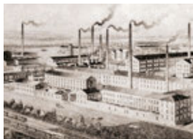
FIRST MECHANICAL FACTORY FOR SANITARY WARE ON THE EUROPEAN CONTINENT, ZNOJMO
